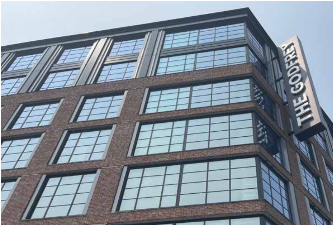
The Godfrey Hotel Detroit is a 227-room boutique hotel in the city's historic Corktown neighborhood. The $2.4 million worth of sheet metal work the hotel required was done by SMACNA Detroit member CASS Sheet Metal.
