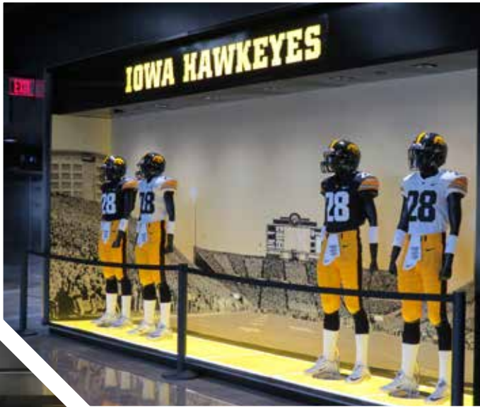
LEFT & RIGHT: The new concourse areas contain 16 gage carbon steel wall panels with 3/16" thick polished stainless steel frames and trim at backlit graphic display panels in
