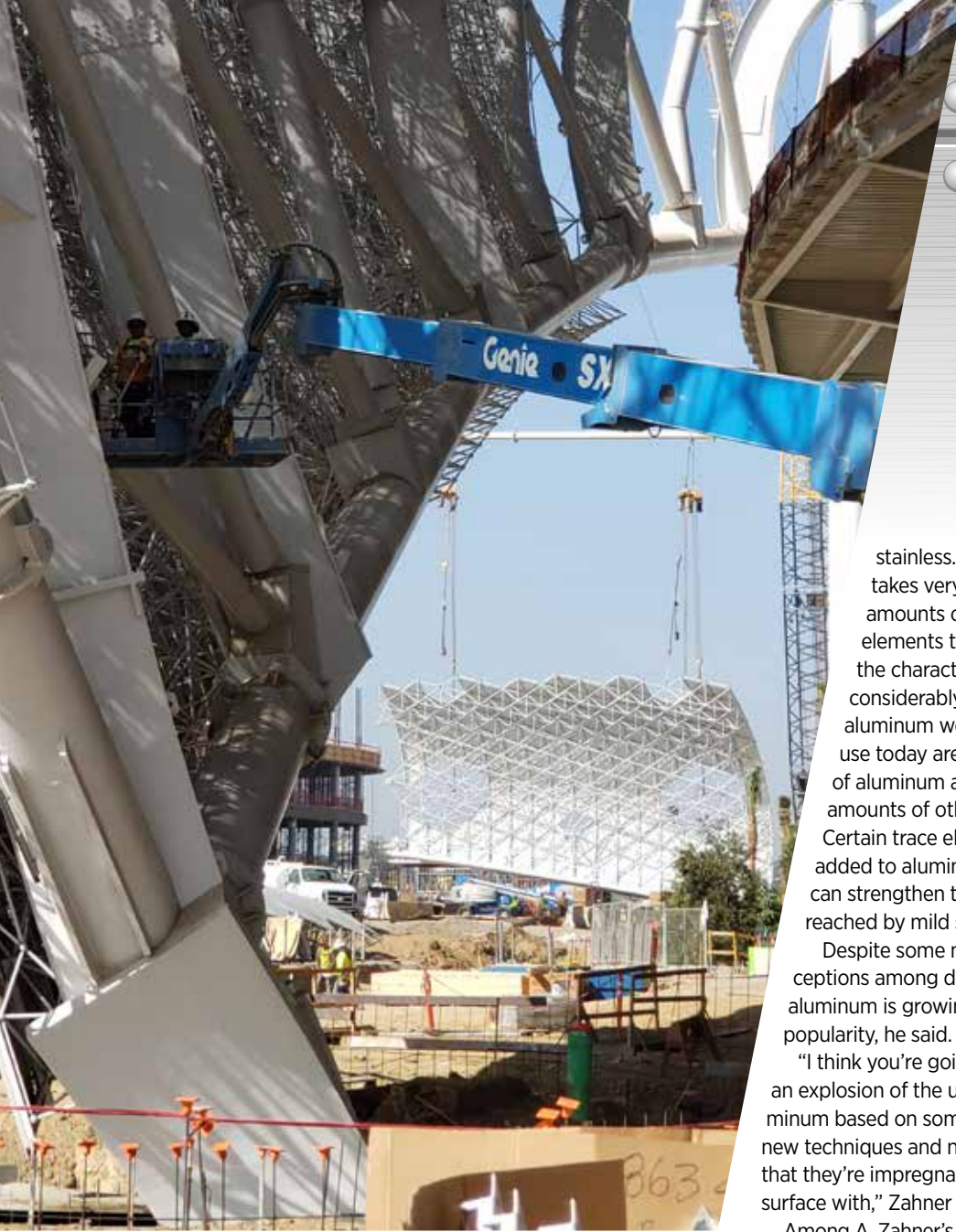
LEFT: SoFi Stadium in Inglewood Calif., home to the L.A. Rams and L.A. Chargers, has 789 perforated, custom white anodized aluminum exterior panels that were manufactured by A. Zahner.
