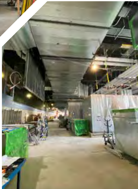
RIGHT: An AHU-604 (front) and AHU-603 (back). The overhead ductwork in front is 88x56 supply air, 4" pressure class and 4" liner.
