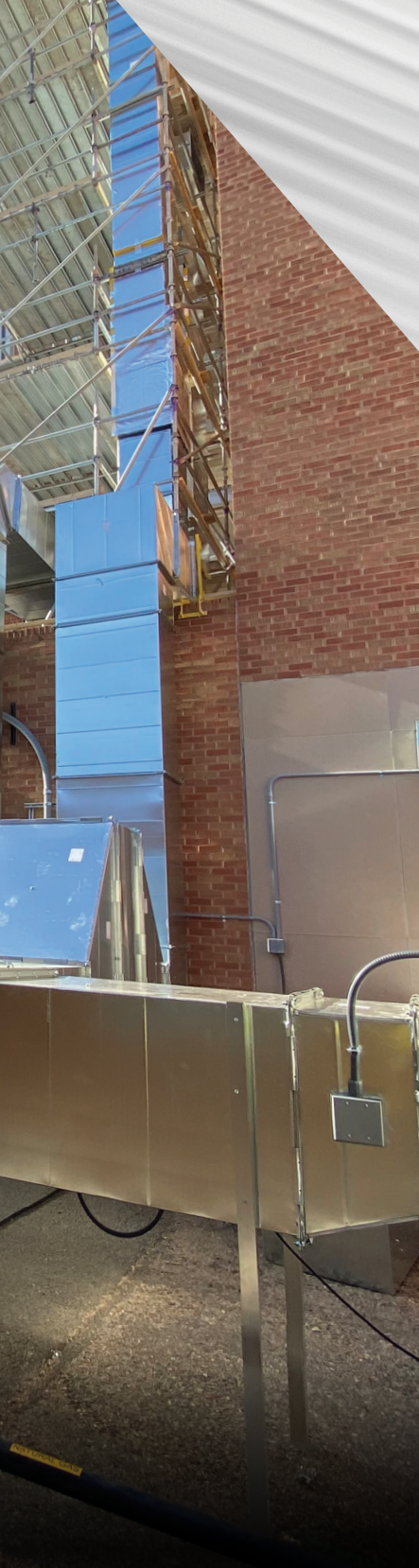
Ductwork installed by CSM runs along the exterior of St. Mary-Corwin Medical Center in Pueblo, Colorado. Two floors of the hospital were converted to negative pressure rooms for COVID-19 patients.
