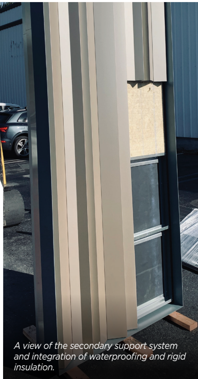
The GES Sheet Metal project team with DPR construction observes a close-up review by the architects. A section of the mock-up has been cut away to allow the design team to see the materials used inside the metal panel.
