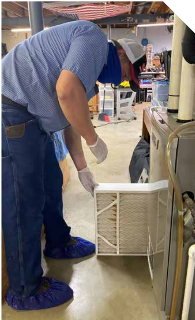
BELOW: A Welsch employee performs maintenance and changes a media filter.
